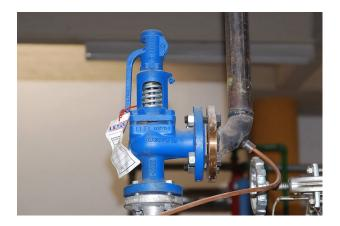
Safety valve prevents overpressure in a vessel or pipe
